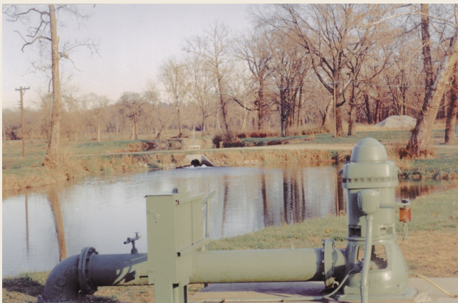
High-capacity turbine pump installed on a municipal well at Rohrsers Island. Recharge lagoon in background. (Photograph by Brent Means, U.S. Geological Survey.)
